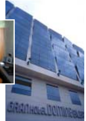
Directly across from the renowned Guggenheim Museum Bilbao
